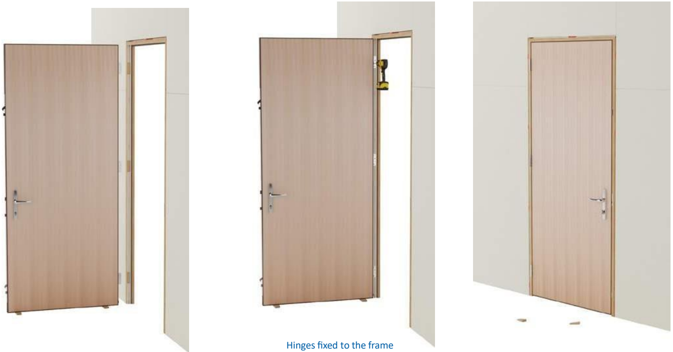
Leaf with hinges fitted is lined up with Leaf operation tested and gaps checked hinge recesses in frame using wedges
