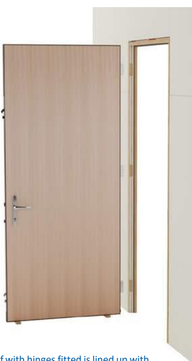
Leaf with hinges fitted is lined up with hinge recesses in frame using wedges
