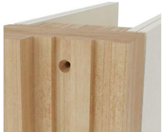
Counter-bored pilot hole in intumescent seal groove
